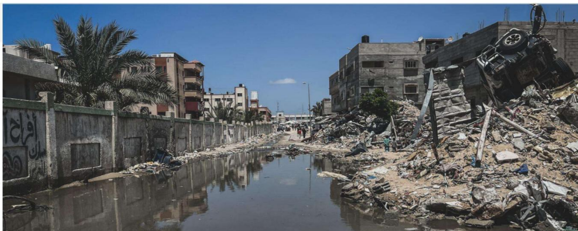
Sewage floods the streets in Khan Younis on May 13, 2024. The decimation of vital infrastructure, including water and sanitation, has raised the risk of diseases in the Strip. | Palestine 2024 © Ben Milpas/MSF
